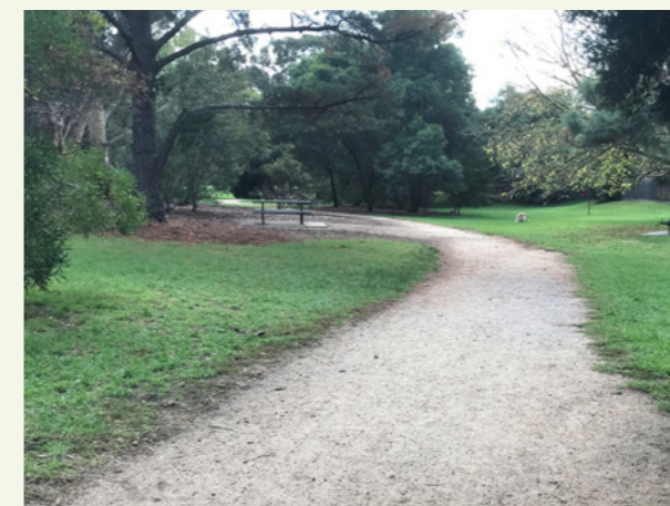
3m wide path with unsealed gravel surface and potential for composite edging where required
