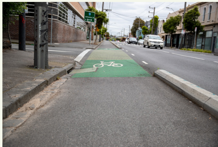
Example of protected bicycle lane treatment on approach to an intersection in Collingwood, Victoria.
