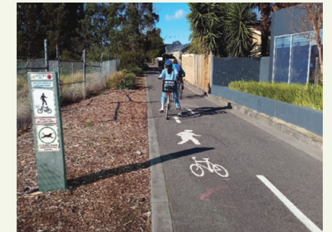
Formal shared path with potential for conflict between bicycle riders and pedestrians
