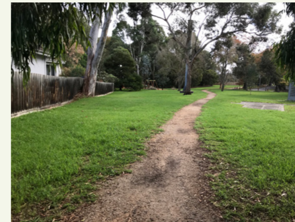
Narrow unsealed path susceptible to safety and drainage issues
