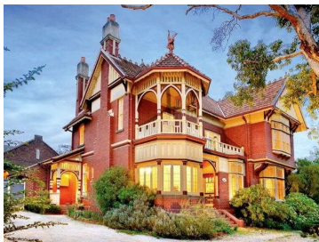
169 Canterbury Road, Canterbury (HO377)
