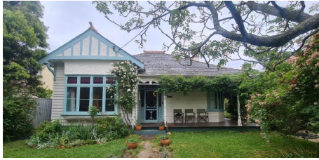
Figure 2 50 Fitzgerald Street photo
