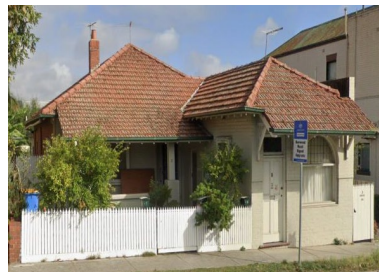
169 Canterbury Road, Canterbury (HO164 precinct)
