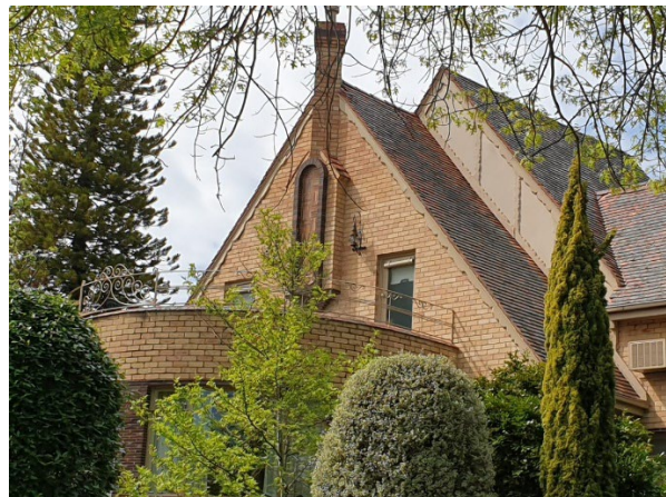
Figure 5 Gable end detail above protruding semi-circular room showing chimney set on 45 degree angle and fine brickwork detail. (Source: GML 2021)
