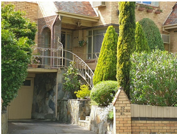
Figure 4 Detail of curved entry steps showing cladding to retaining walls and sub basements walls and mild steel balustrade. (Source: GML 2021)
