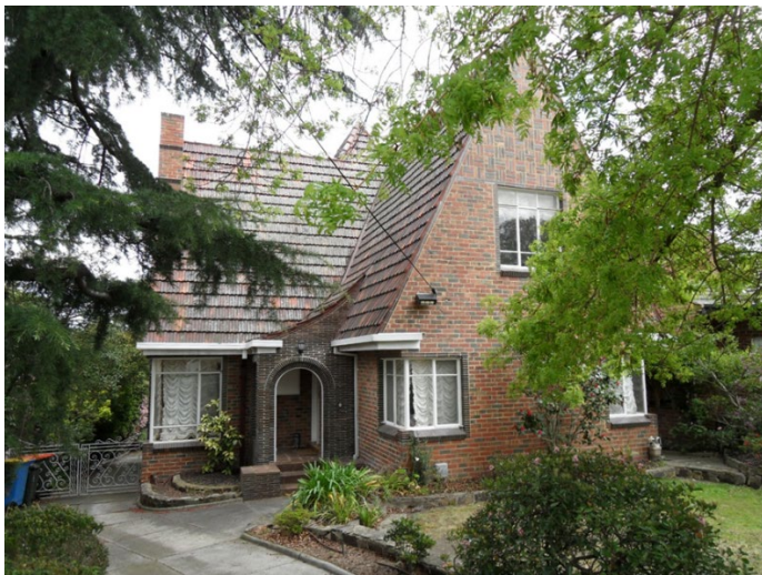
Figure 12 'Vedere', 44 Panoramic Road, Balwyn North, constructed in 1947 (assessed as significant in this study). (Source: Context 2017)
